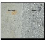
Before and after shot blasting...the profile after should be a little rough. We should discuss with the contractor and make sure that we get the largest machine possible for the project...ask the question as this will impact your schedule if you allow a small machine on site...a small machine is 9"...a good size should just be able to fit through the door.
